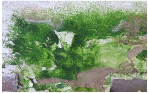
Fig. 1. Detail of the facade of the building with clearly visible biocorrosion
